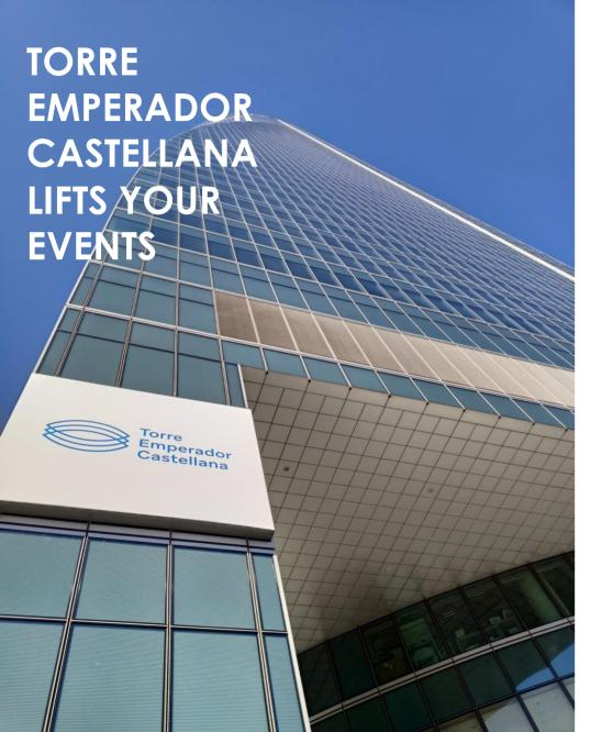
This building is one of the highest skyscrapers in Spain, with a height of 235 meters distributed in 57 floors coated with a double façade sistem, for a thermic and light conditioning isolation of the highest quality.
